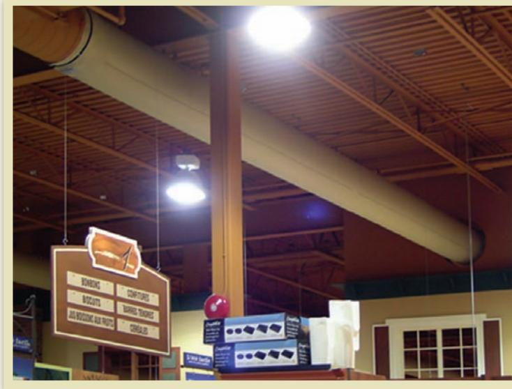
All the components of the heating system, which are major contributors to LEED accreditation for example, are readily available and cost-effective via paybacks even if energy incentives aren't available. The store space heating consists of a wall-mounted solar thermal system, fabric ductwork by Ductsox Corp, and heat recovery by a Compressor Systems Control (CSC) system. Air conditioning is handled by a conventional high-efficiency air handling system and uses the same fabric ductwork system.
