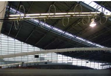
Metal duct also would have needed hundreds of registers, which have proven less effective in even air distribution. Instead of registers, the DuraTex fabric has factory-engineered permeability to distribute up to 15 percent of the airflow through the material. The remaining 85 percent of air distribution is through hundreds of CAD-engineered perforations that run the entire lengths of the convention center's ductwork. The
