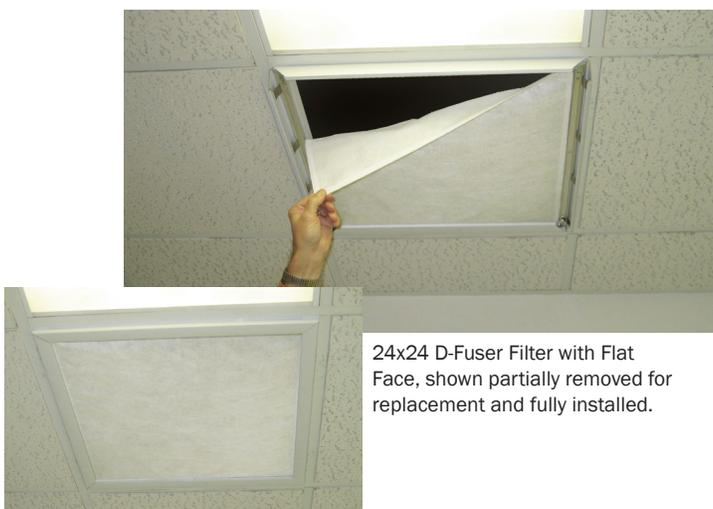
24x24 D-Fuser Filter with Flat Face, shown partially removed for replacement and fully installed.
