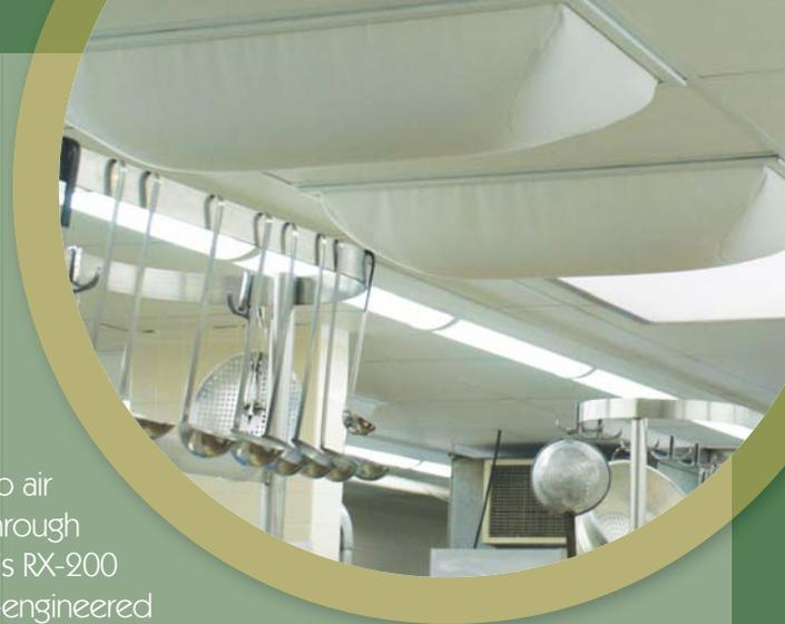
Make-up air flows through LabSox's RX-200 factory-engineered fabric at a low velocity of 70 to 95-fpm. The end result is a slower, more even airflow distribution that allows the kitchen exhaust hoods and other exhaust outlets to perform correctly.
