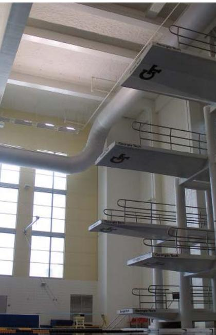
In addition to saving material and labor costs, fabric duct doesn't require interior insulation and exterior epoxy coatings to prevent condensation and corrosion respectively, that's inherent in natatorium environments. "Fabric duct offers a bonus over metal in natatorium environments, because pool chemicals do not degrade polyester fabric material," said Saunders.
