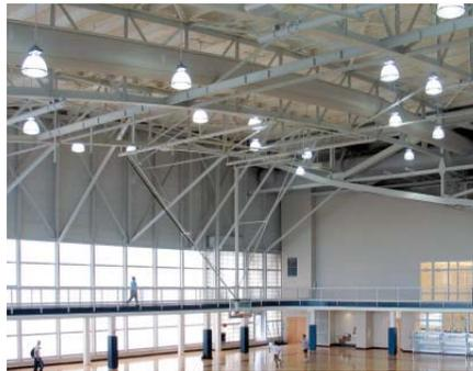
Sedona fabric duct with Comfort-Flow air dispersion and linear vents manufactured by DuctSox, Dubuque, Iowa, helped cut both material and installation costs. Gray 56-inch-diameter fabric duct distributes dry, conditioned air along a wall of exterior windows and three 36-inch-diameter ceiling-hung branches span the entire width of the pool surface. A
