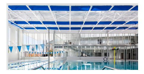
fabric composition that allows for the entire duct to act as a diffuser, which eliminates hot and cold spots and creates an evenly distributed airflow. Fabric ducts also absorb sound, unlike metal.
