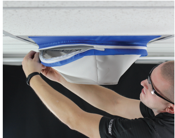
Zipping the Displacement Panel to the Perimeter Panel
