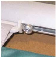
Attach the Tension Clips of the fabric to the Tensioning Basket. Complete the connection by zippering the duct to the Inlet Belt.
