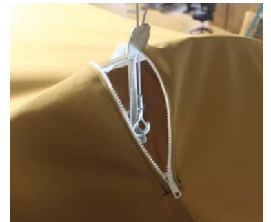
12:00 top zipper of the Elbow to insert the Direct Hang Cable Drop
