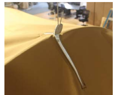
Grommet at the end of the Elbow to insert the Direct Hang Cable Drop
