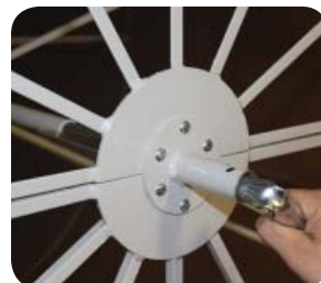
Interior Section ITR Tensioning
