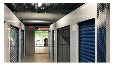
Working closely with DuctSox engineers, Morningstar implemented a custom fabric ductwork system for Summerville. The facility's existing metal ductwork, which spanned several hallwavs between units, was replaced by several rows of grey fabric ductwork suspended from the ceiling. Significantly, the fabric duct was mounted above storage units, rather than down various hallways, to improve airflow above customer's property and boost the facility's environmental control. This clean.
