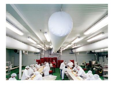
Technology advancements in fabric have created an opportunity for DuctSox to be used in applications where there are specific performance requirements. Anti-static fabrics are ideal for data centers and anti-microbial treated fabrics for laboratories, food processing and grow facilities.
