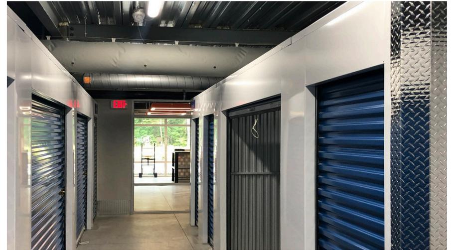
Working closely with DuctSox engineers, Morningstar implemented a custom fabric ductwork system for Summerville. The facility’s existing metal ductwork, which spanned several hallways between units, was replaced by several rows of grey fabric ductwork suspended from the ceiling. Significantly, the fabric duct was mounted above storage units, rather than down various hallways, to improve airflow above customer’s property and boost the facility’s environmental control. This clean,
