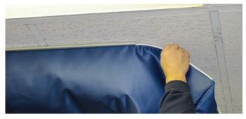
**Step 7**Tighten cleats. Pull cord tight and lock in cleat.
