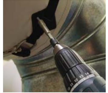
Slide Glider attachments of the DuctSox into the U-track bottom channel. Unzip fittings and slide them in place independently of the straight sections. Close all zipper connections before moving to Step 5.
