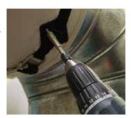
Slide Glider or Cord-In attachments of the DuctSox into the U-track bottom channel. Unzip fittings and slide them in place independently of the straight sections. Close all zipper connections before moving to Step 5.
