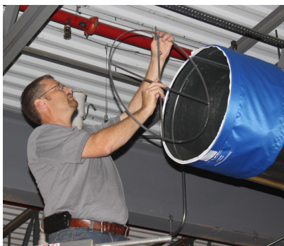
Install Universal Ring Assembly on Cable
