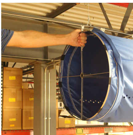
Pull back on Tensioning Basket
