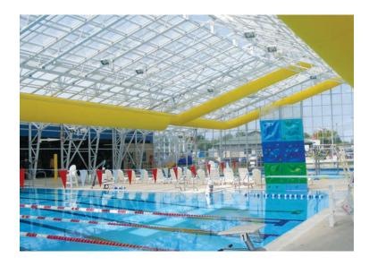
ystems that utilize fabric, such as DuctSox, provide targeted, precise and efficient air dispersion for new construction and retrofit projects. Additional benefits include a total lifetime ownership cost that is significantly less than a comparable metal ductwork layout and the ability for a system to be custom designed based on the application.
