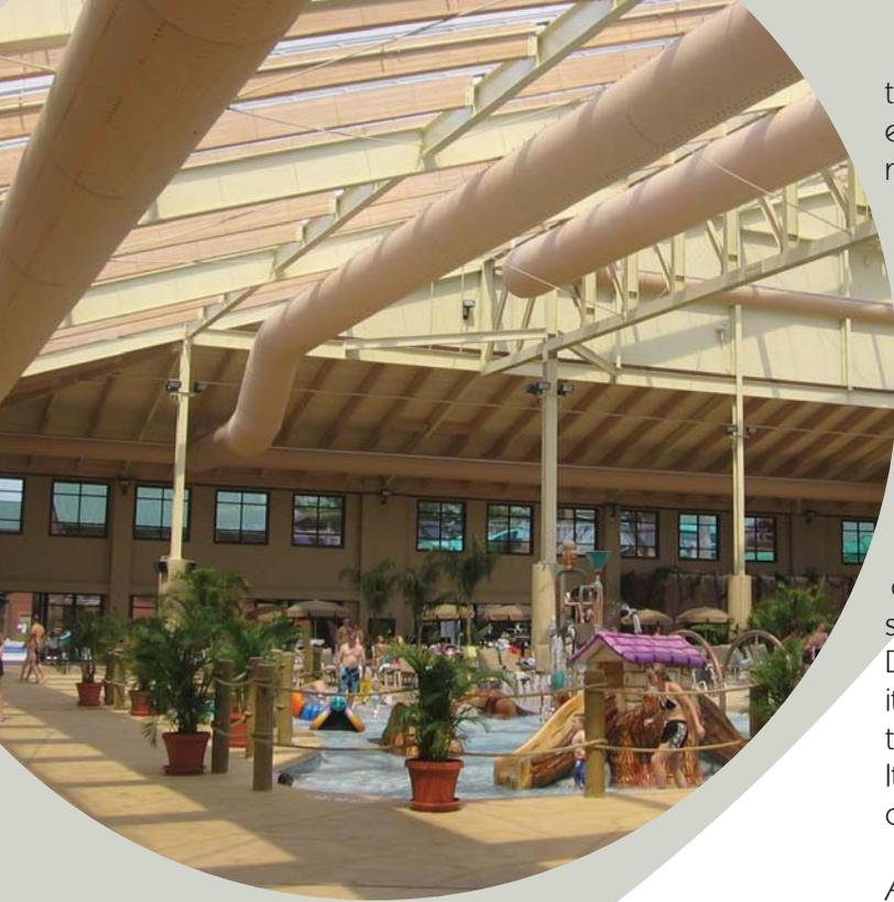
around six 120-foot long runs of 60-inch-diameter TuffTex commercial grade fabric duct have a variety of orifice diameters ranging from 3/4-inches to 1-1/2-inches and duct circumference placements. The two 19-foot-high perimeter runs have two linear arrays of orifices directed toward the windows and another array towards the deck.
