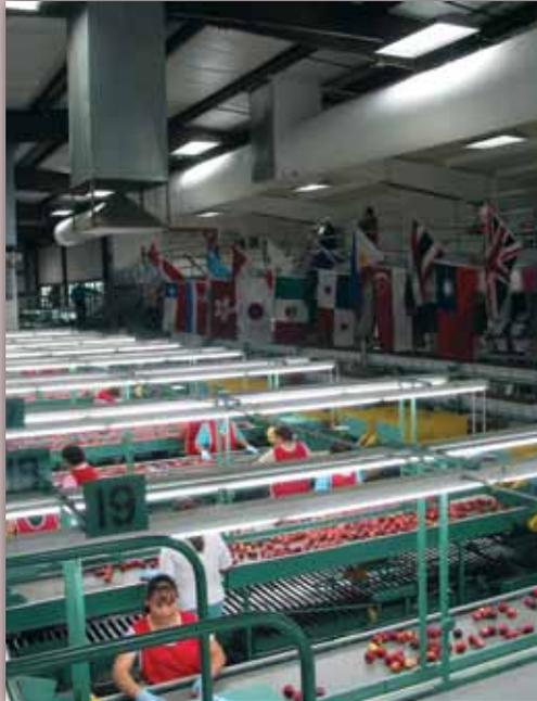
Instead, Chapman specified TuffTex premium fabric duct with a High-Throw airflow from DuctSox, Dubuque, Iowa. Marcelo Carino, salesman at manufacturer's representative, Air Tech Sales, Roseville, Calif. helped Chapman with the DuctSox design. The streamlined ductwork has linear diffusion in the form of DuctSox's high-throw orifices running the entire length of the mezzanine, which produces a more even airflow than registers mounted on metal duct every 10 feet.
