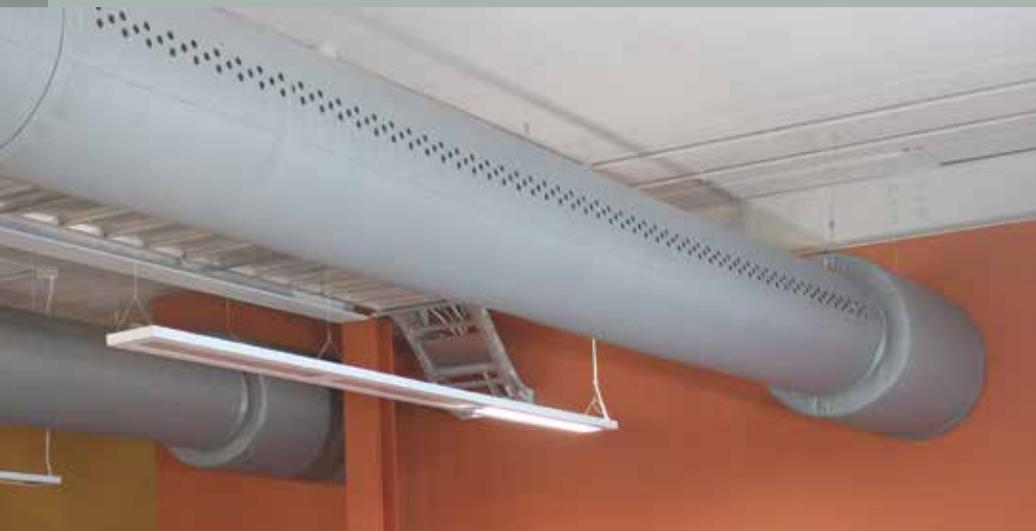
with just a turn of a wrench for wrinkle-free aesthetics. The result is fabric duct that appears inflated regardless of AHU operation or air pressure, which add to the office areas' aesthetics.
