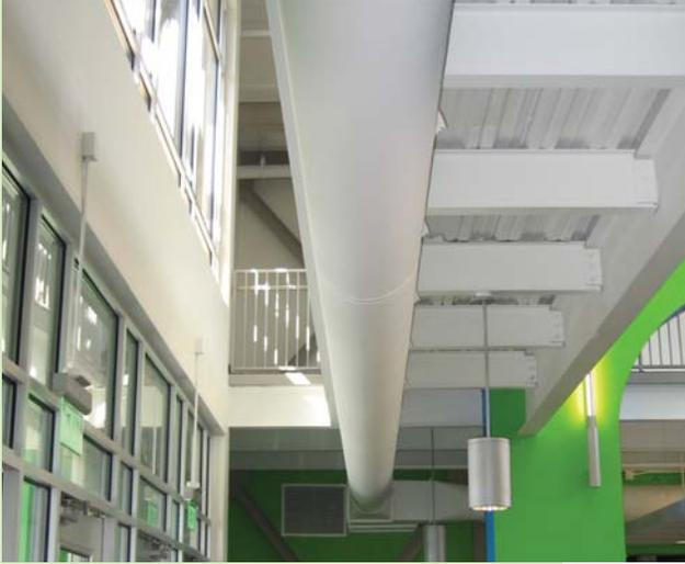
Traditional round fabric duct by DuctSox Corp.
