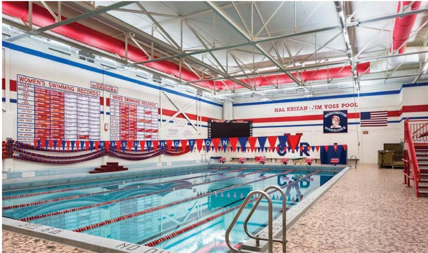
Fabric duct reduces ventilation material/installation costs and fast-tracks installation time by 60% to assure work completion during a short two-month summer recess. Shive-Hattery specifies fabric duct more frequently today, but now incorporates the industry's latest innovations such as linear L-vents for indoor air comfort, custom colors to match school colors, in-duct tensioning systems for 24/7 inflated aesthetic appearance and other improvements.
