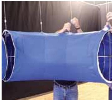
Attach Direct Hang Cable Drops to assembled elbow.
