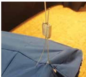
Slit at the end of the Elbow to insert the Direct Hang Cable Drop
