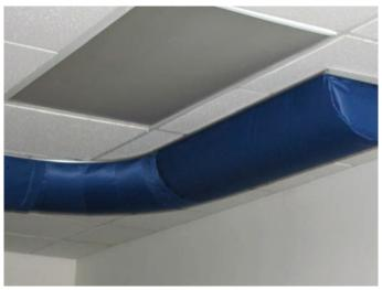
**Step 7**Tighten cleats. Pull cord tight and lock in cleat.
