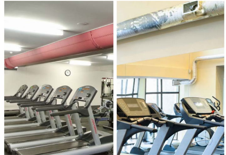
DuctSox shown on left requires minimal exterior maintenance vs metal system shown on right that will require high maintenance costs to repaint and repairs dents.
